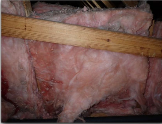
Insulation on vertical attic walls
