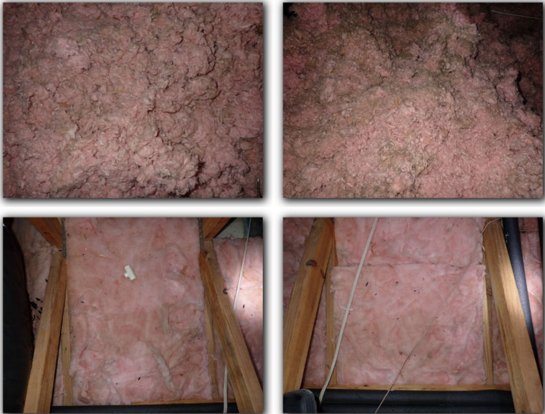
Insulation on horizontal areas
