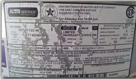
Water Heater Manufacturing Date
