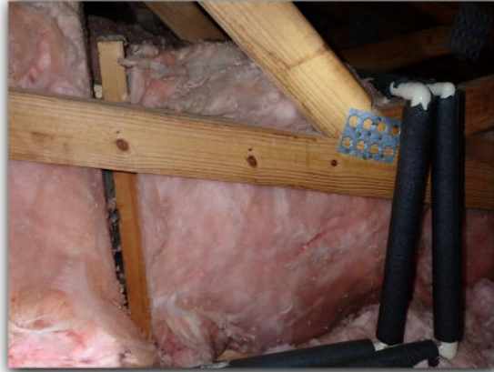
Insulation on vertical attic walls
